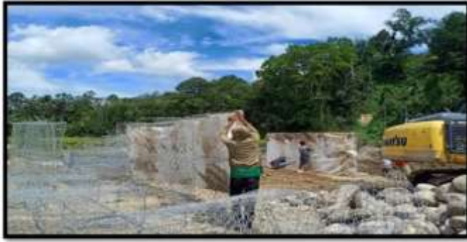
Figure 1. Gabion installation phase showing geotextile underneath the baskets
